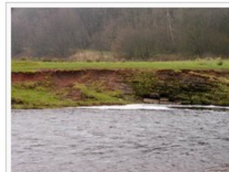
Liddel Motte bend reinforcement © Howard Mattinson
