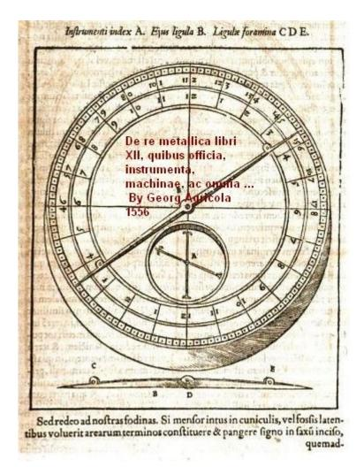
The compass is used for bearings, and measurement of a angles. Angles can be adjusted to total the proper degrees after survey.
